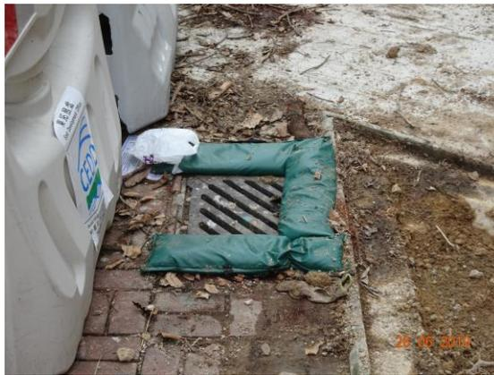
Sand bags was provided for the existing gully to prevent loose material flushing inside during rainstorm.
