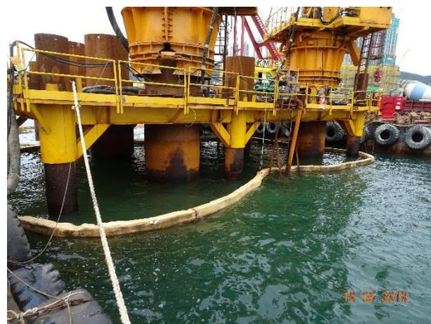
Silt Curtain was provided for the bored pile working platform.
