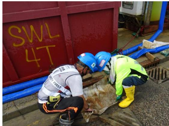
Geotextile was installed in the existing gully to prevent loose material flushing inside during rainstorm.
