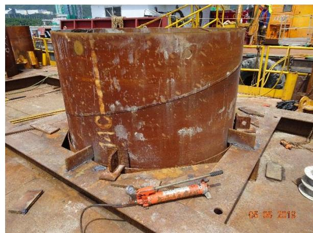
Cofferdam was used during marine bored pile work.
