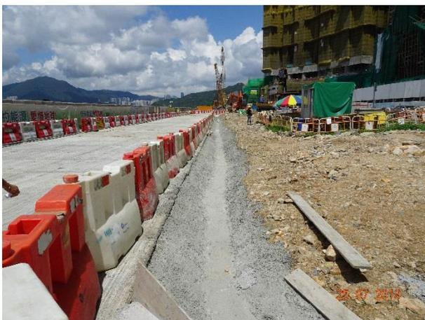
Part of the temporary drainage was installed to divert the site runoff to the de-silting facilities.
