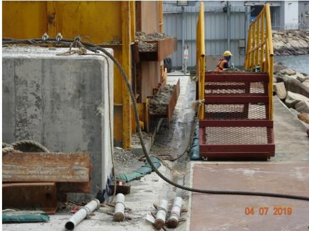
Earth bund was provided at the site boundary to prevent muddy surface run-off leakage into the water body.
