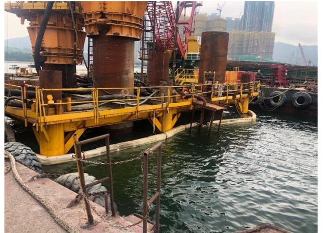
Silt curtain was installed to prevent the muddy water leakage into the water body.
