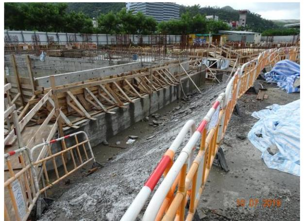
Concrete the exposed surface to reduce to create muddy water during rainstorm.
