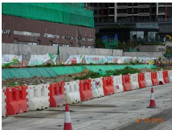
Using tarpaulin cover the exposed area to prevent generate turbidity runoff during rainstorm.
