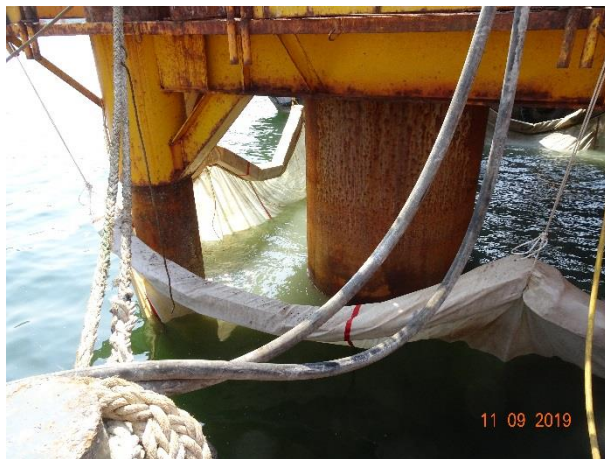
Silt-curtain had been provided to prevent muddy water overflow from the piling platform.
