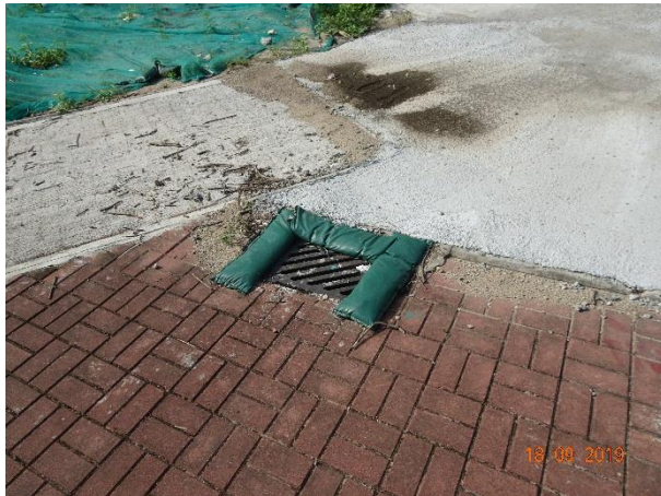
Sand bags had been provide to prevent site runoff overflow to the existing manhole.
