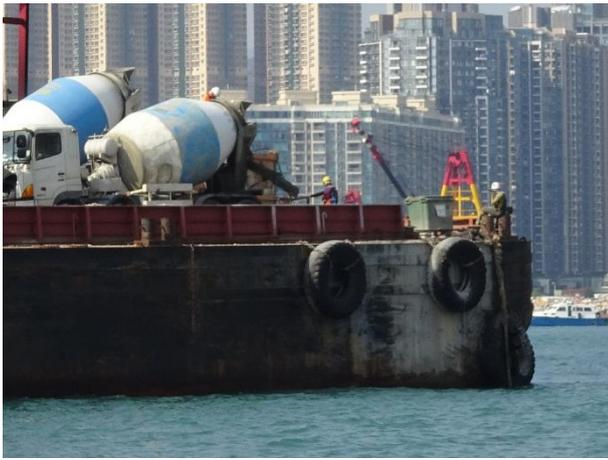
Waste skip was provided to storage the concrete washing water during concreting work.
