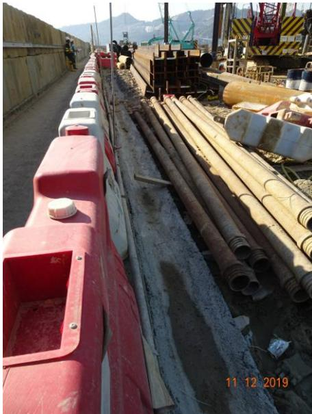
Trench had been installed beside the sea front to prevent muddy surface run-off overflow during rainstorm.
