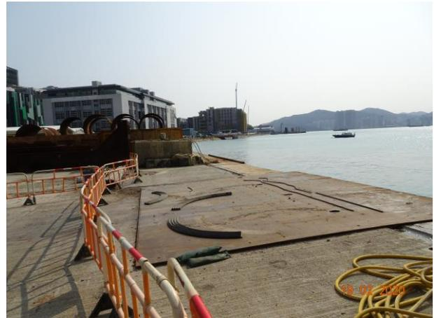
Temporary trench had been installed at the sea fount to prevent muddy run-off overflow into the water body during
