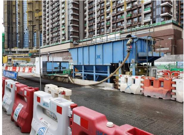
Treatment facilities was installed at site to treat the site generated water prior discharge.
