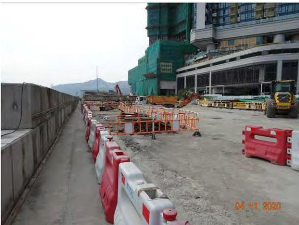
Trench had been installed beside the sea front to prevent muddy surface run-off overflow during rainstorm.
